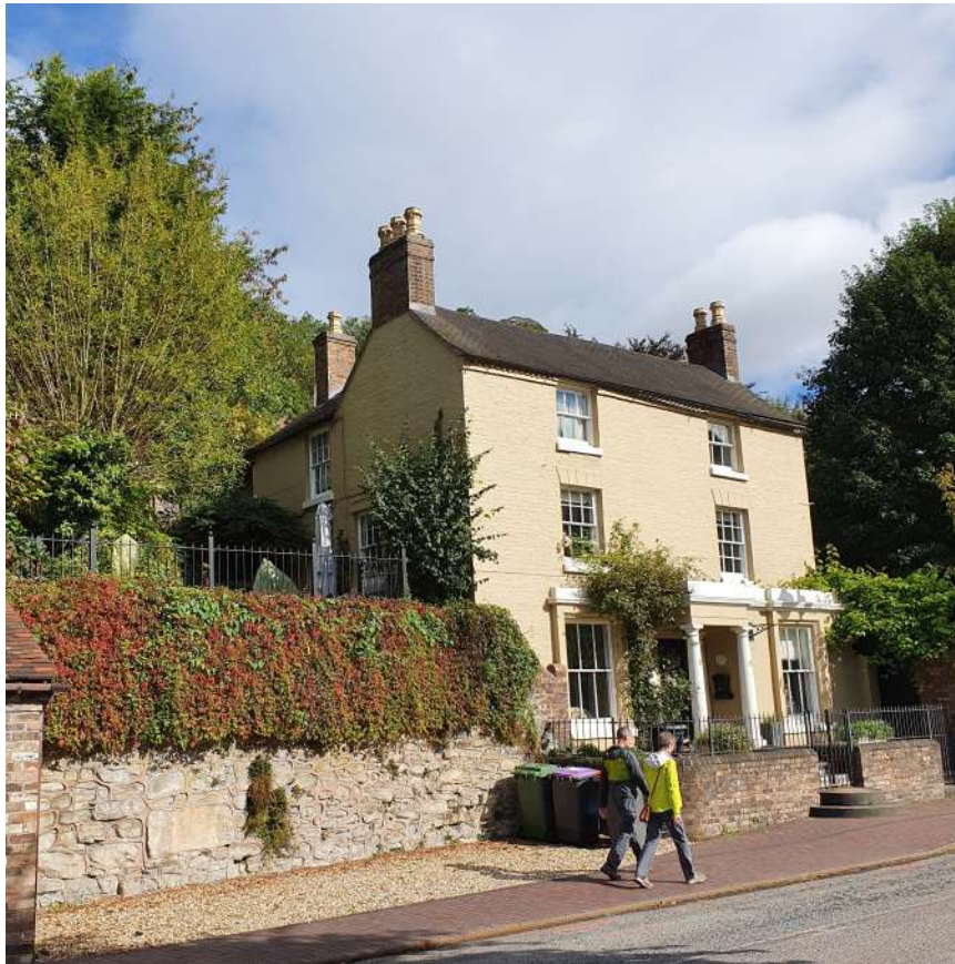
Figure 8: The Wharfage, Grade II Listed Building
