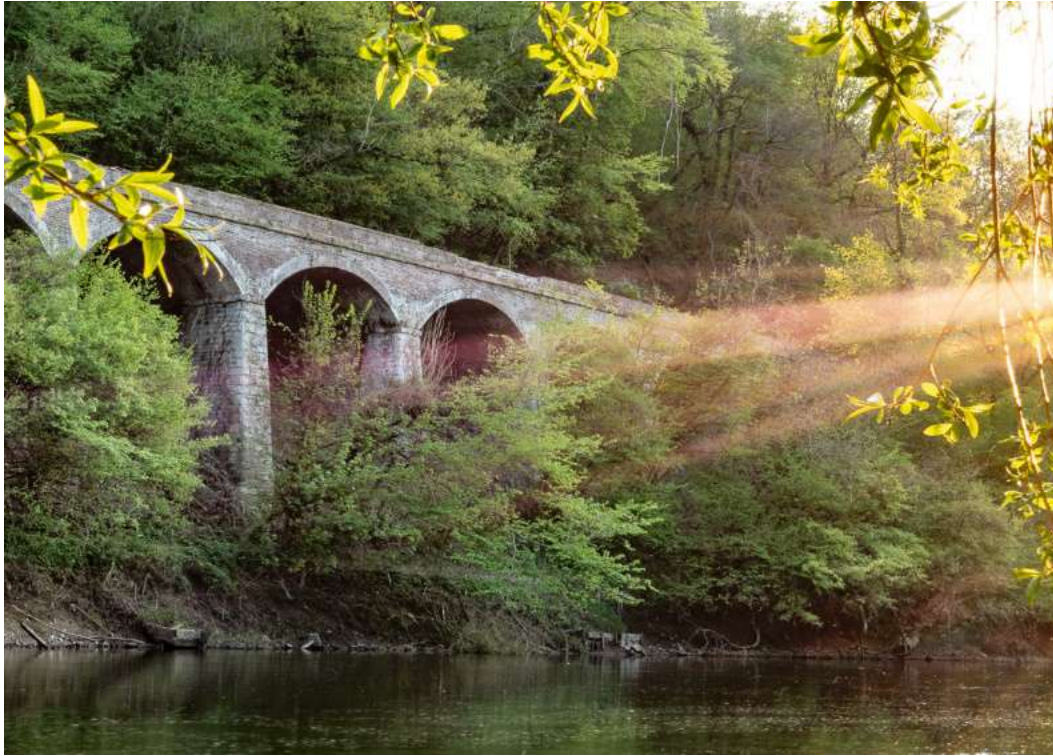
Figure 13: Viaduct at Coalbrookdale
