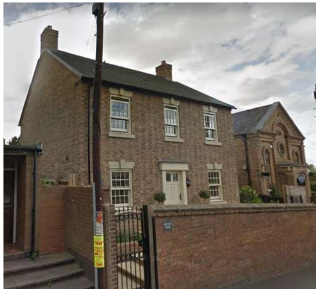
Figure 18: Building set in line with existing buildings with brick boundary wall to edge of street. Using a good brick match for adjacent historic building, sympathetic roof pitch, chimney stacks, sash windows, six panel door with door case, boundary wall and iron gate.
